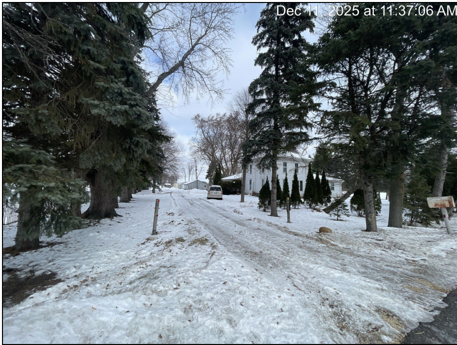
Picture 2: Looking north at the existing structures on the parcel.
