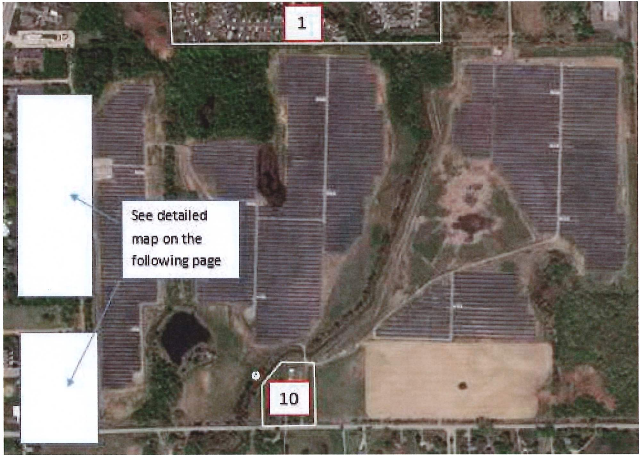
DTE Lapeer Solar Projects - Turrill Adjoining Properties
