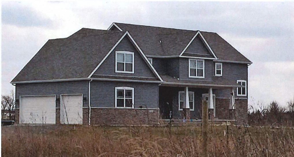
4,255 square foot estate home under construction, adjacent to Portage Solar Farm located in Indiana On-site pond and attached garage (cost estimated at $465,000) April 2018
