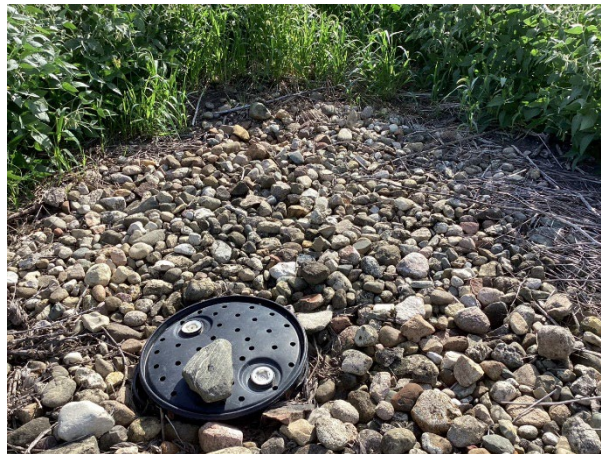
Photo 5: Drain tile at SP-3 within historic AOI 1.
